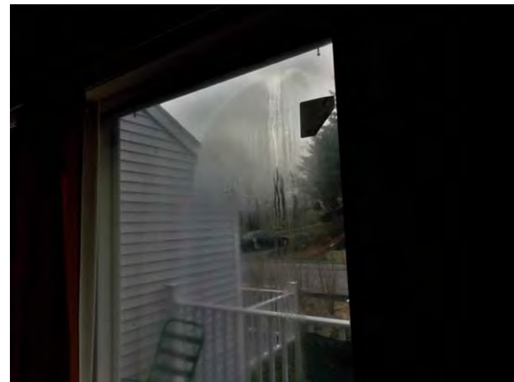
The fogged window indicates possible window seal failure.
