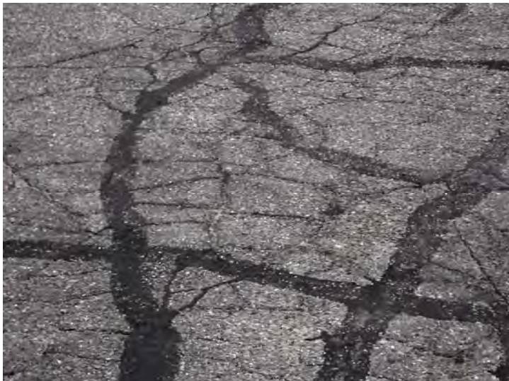
A close-up view of a cracked section of asphalt paving.
