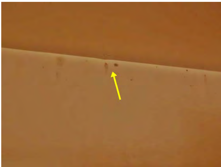
Suspected mold in one of the bathrooms.
