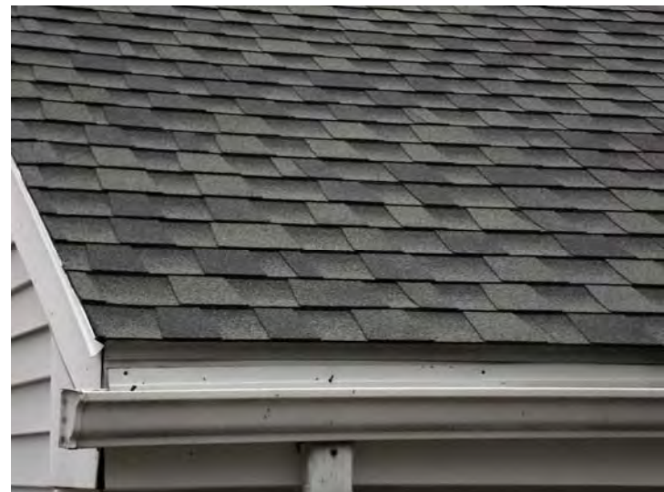
The roof coverings have been recently replaced with architectural shingles.
